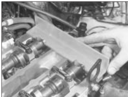
10.10 Fit camshaft aligning tool to ensure engine is locked with Nos 1 and 4 cylinders at TDC
