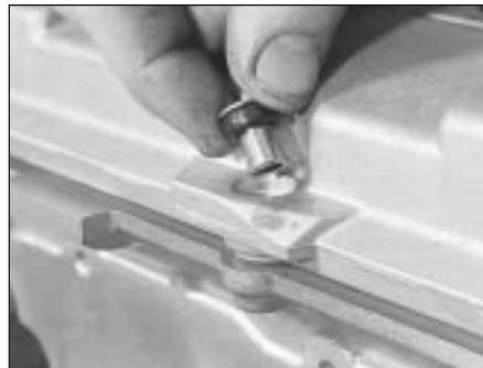
5.9 Ensure rubber seal is fitted to each cover bolt spacer, as shown
